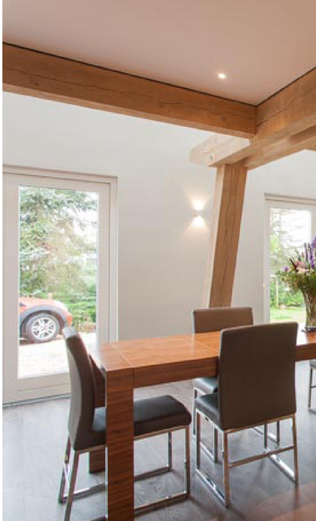
has been custom-made with a matt finish, and an airtight seal was created with the help of expanding foam tape around doors, windows and rooflights.
